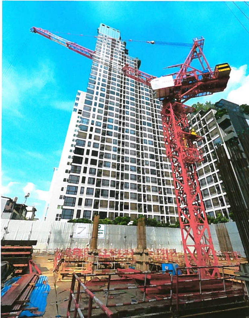
[TC2] NTP QTP160-12T LUFFING JIB TOWER CRANE (S/N: 22-030151-003)
